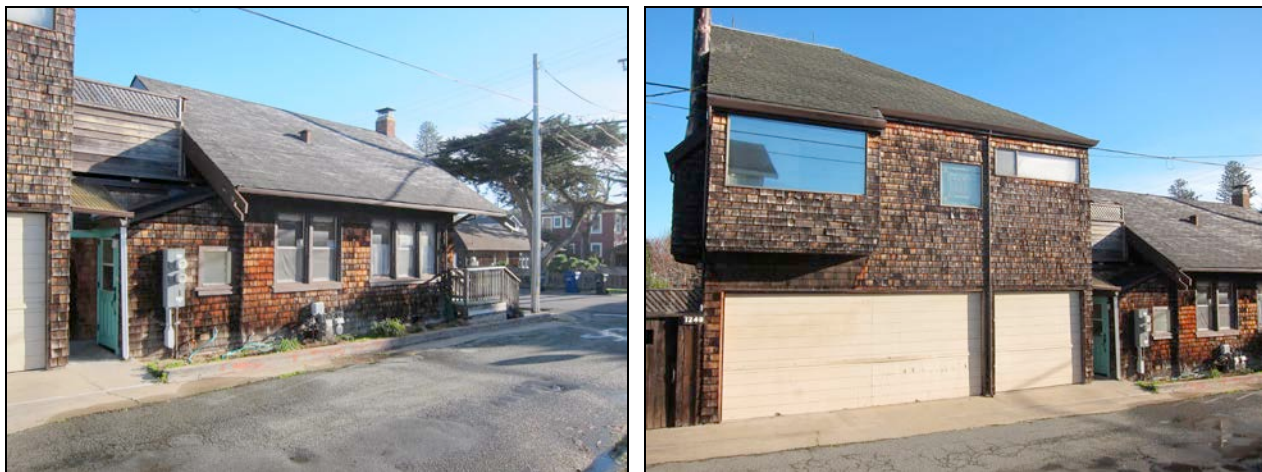
Figures 4 and 5. Left image shows the south (Union St.) elevation of the Craftsman bungalow where it meets the circa-1971 addition. Right image shows the two-story, circa-1971 addition on Union Street.
